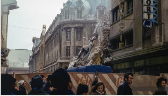
(ABOVE) The last major earthquake (1977) completely destroyed some historical buildings. Experts are expecting another major earthquake in the following decade.
